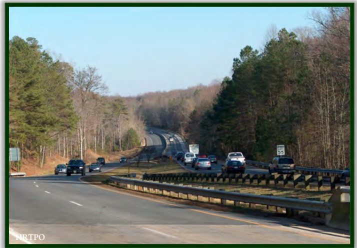
Route 199 in James City County, widened in 2005.
