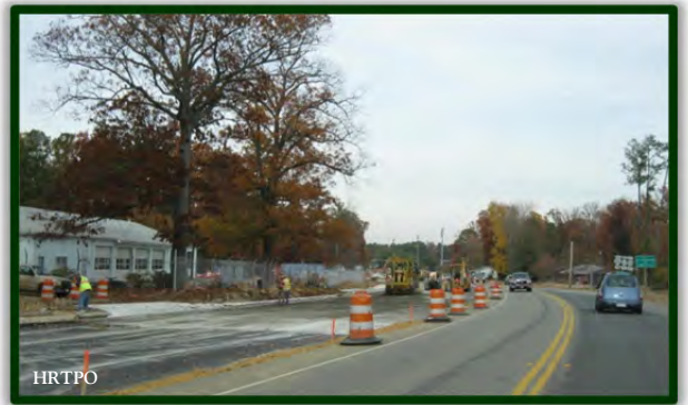
Ironbound Road Construction
