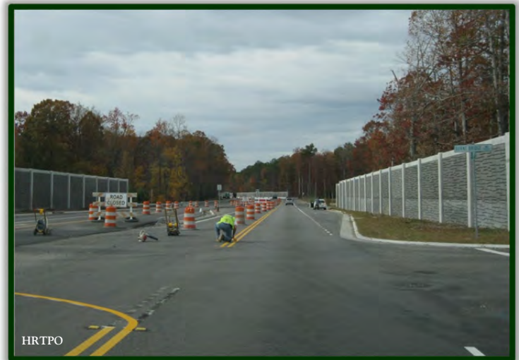
Fort Eustis Boulevard Construction
